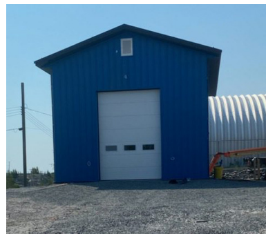
Nouvelle installation de Great Slave Bottling Company's
